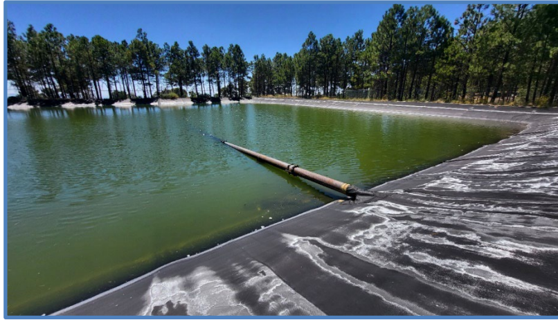
Palisades Administrative Site - Lagoon
