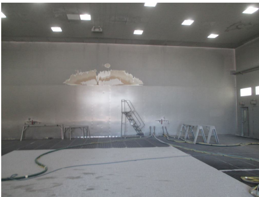
Photo 4: South facing view of the blasting room in the ASF. Blasting media and debris is visible in the center of the floor.
