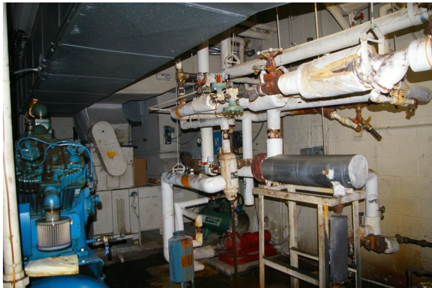
Photo 12: West facing view of the mechanical room adjacent to the high bay area. The pipe insulation in the room was fiberglass.
