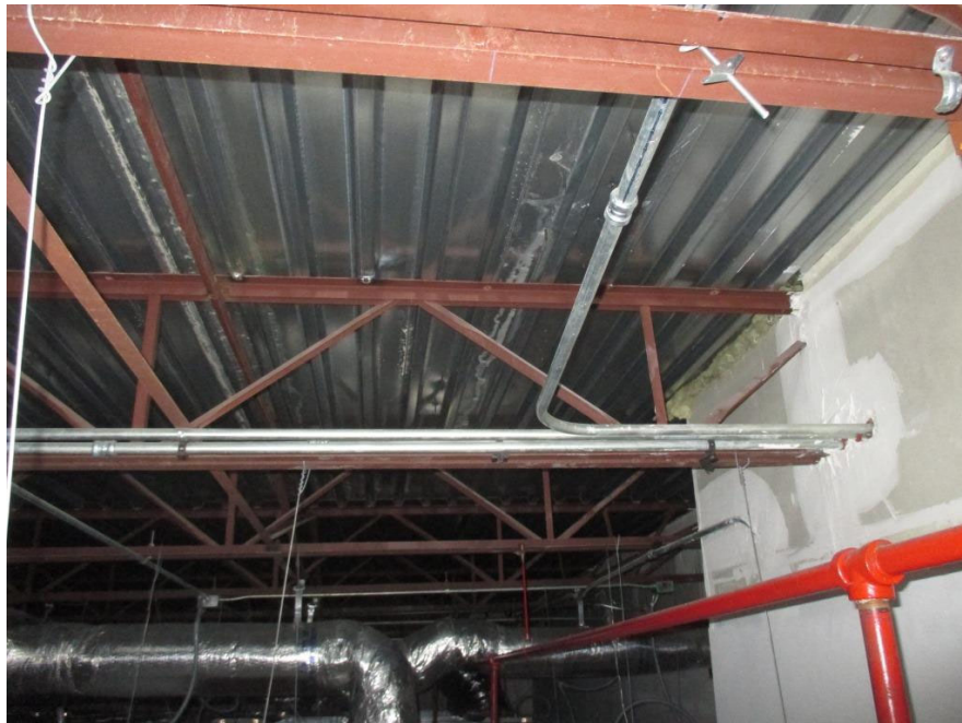
Photo 2: Typical view above the SACT.
