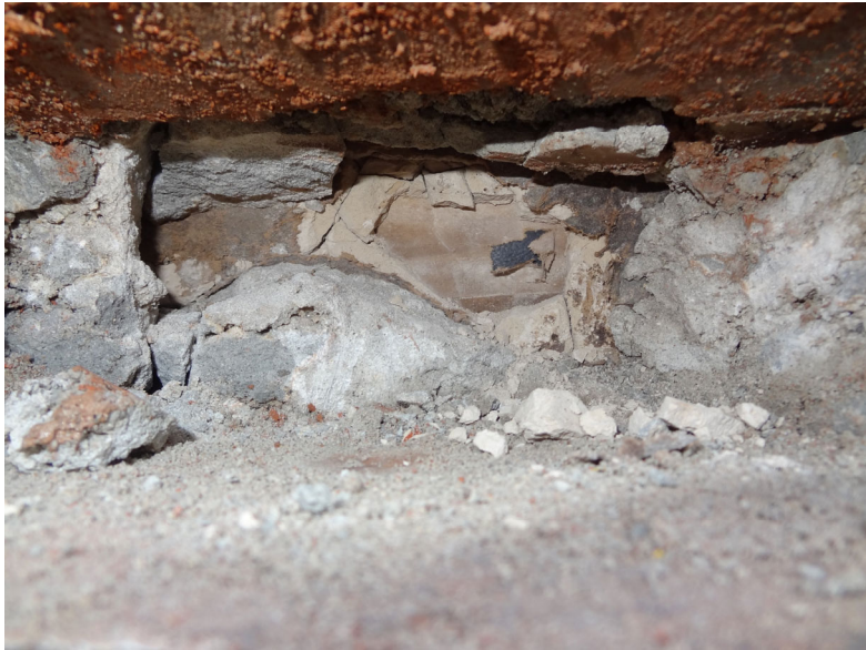
Photo 15: Typical view of gypsum wallboard observed in the high bay wall cavity.
