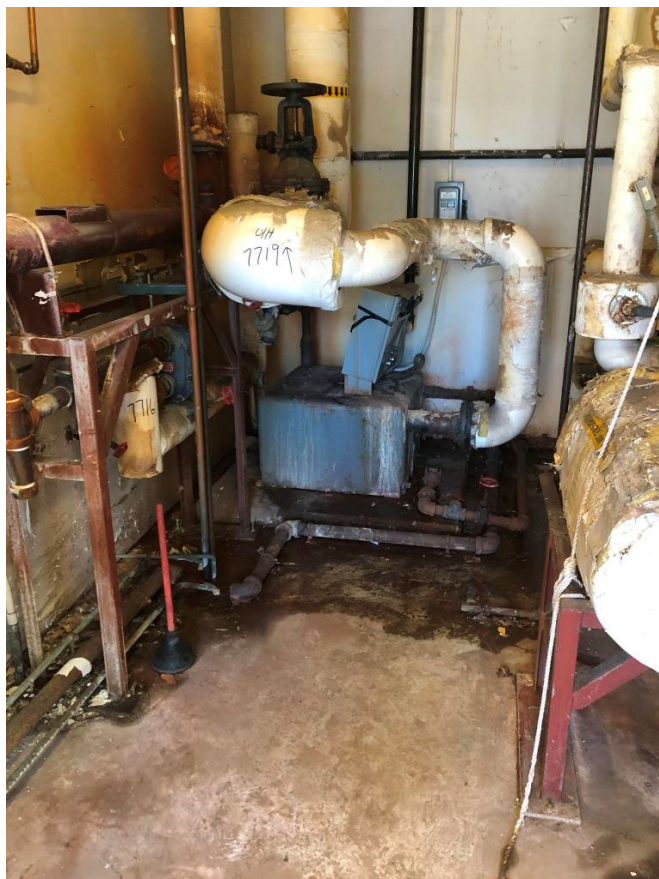
Photo 8: South facing view of the mechanical room adjacent to the blasting room. The insulation in the room was fiberglass.
