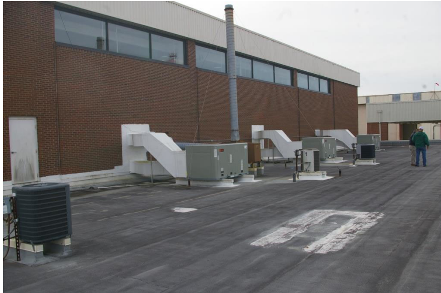
Photo 9: West facing view of the roof on the original building above the classroom area. No ACM was identified in the roof.
