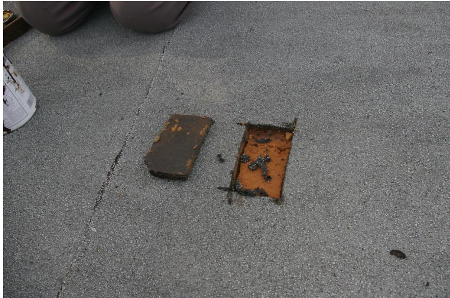
Photo 11: Typical view of a roof cut made on the original building.
