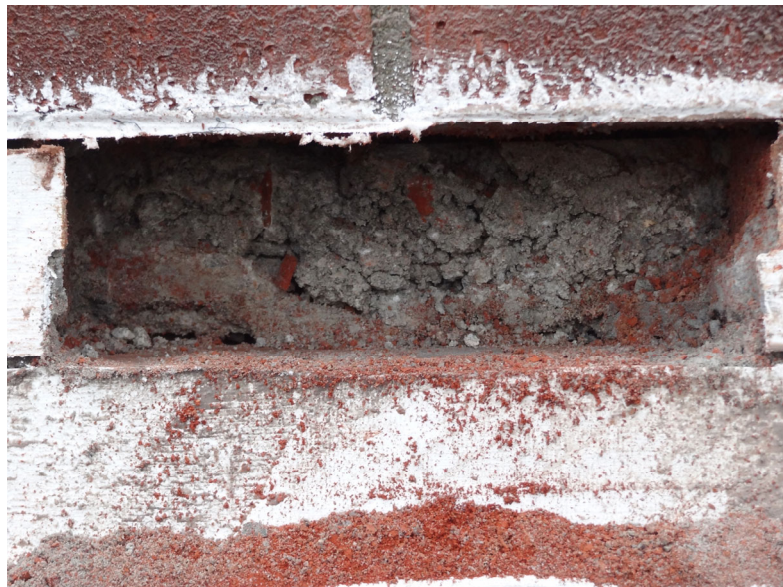
Photo 14: Typical view of the high bay wall cavity at brick removal location B1. No waterproofing material was observed.
