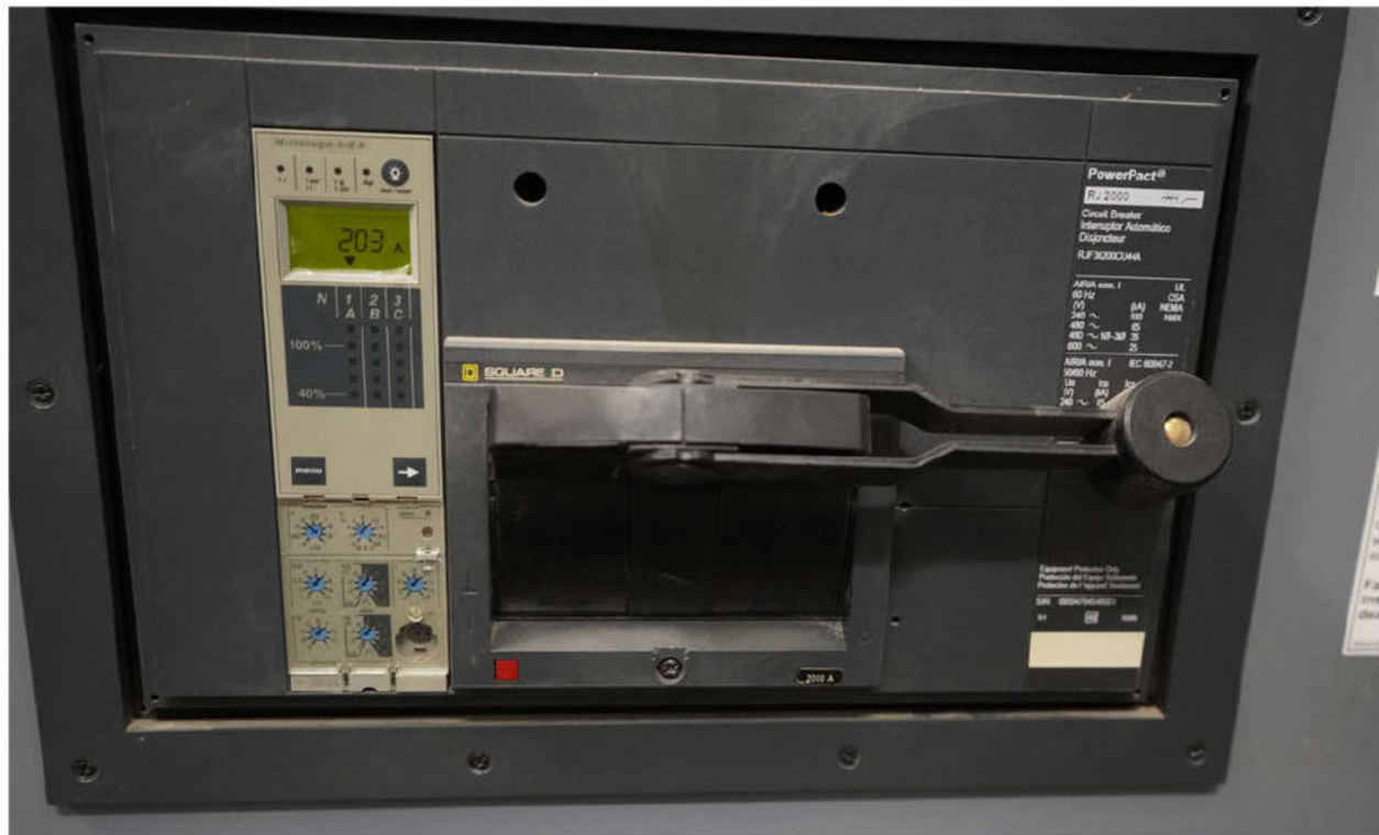
Figure 3-4 Micrologic 6.0A
