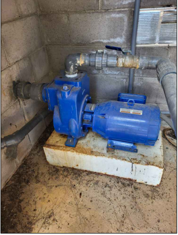
EXISTING 5HP CENTRIFUGAL PUMP WITH 2" INLET/ OUTLET
