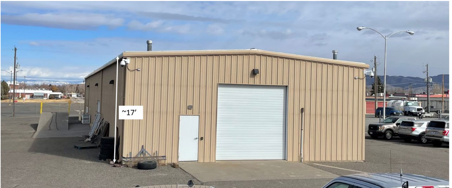
Warehouse Building – Looking North
