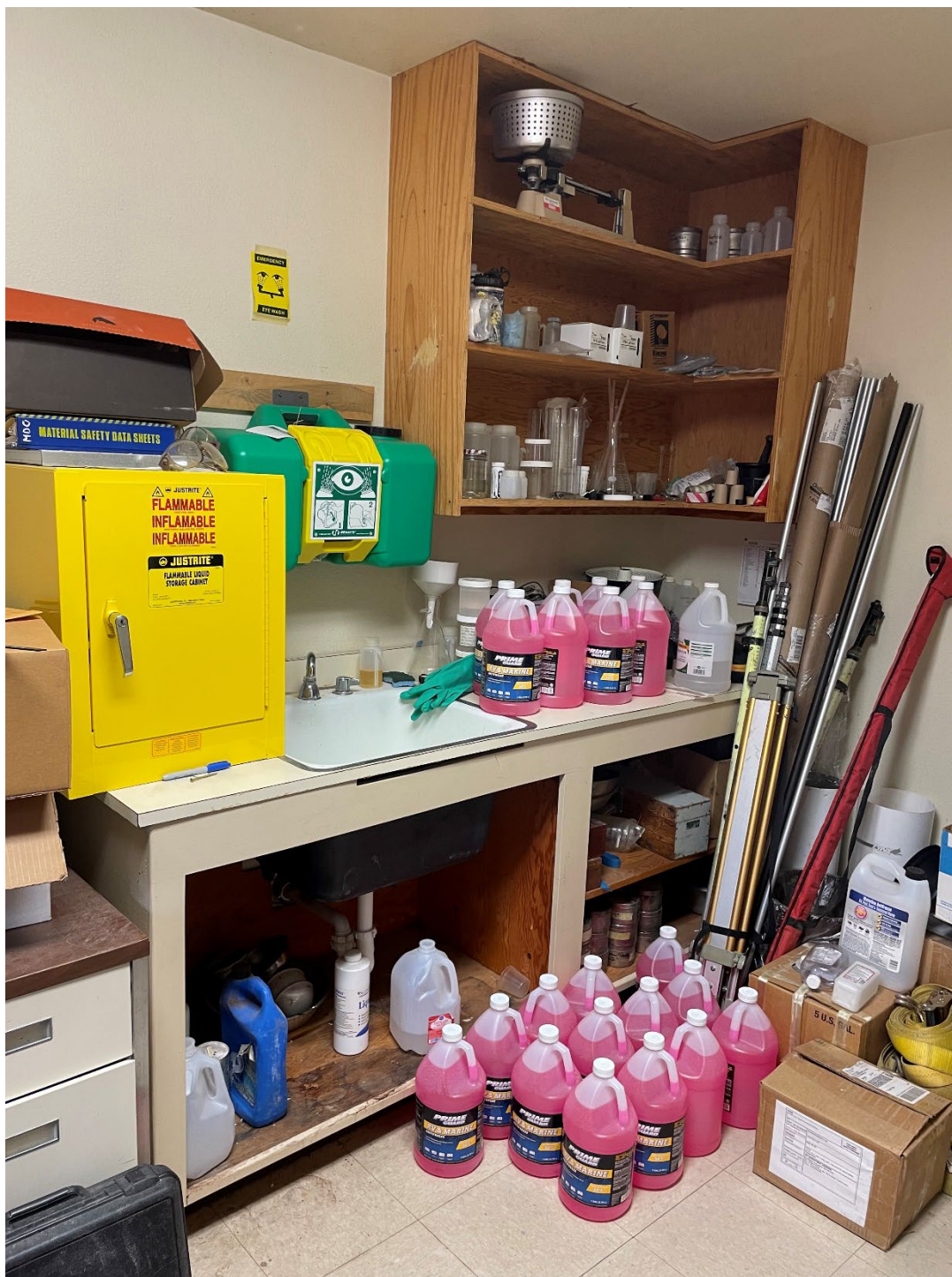
Office 3 sink, countertop, and shelf to be demolished.
