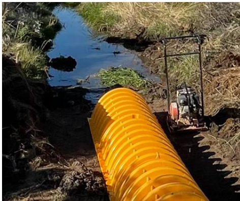
Figure 9: StormTech Chamber Installation
