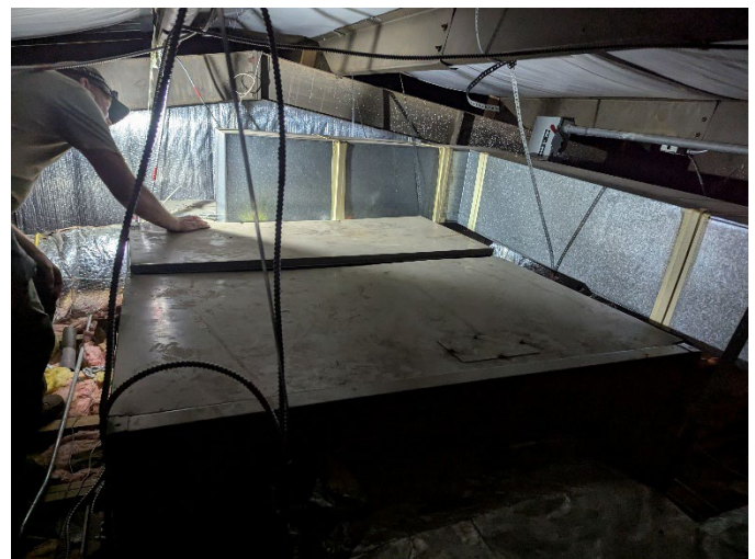
Figure 4: AIR HANDLER.
