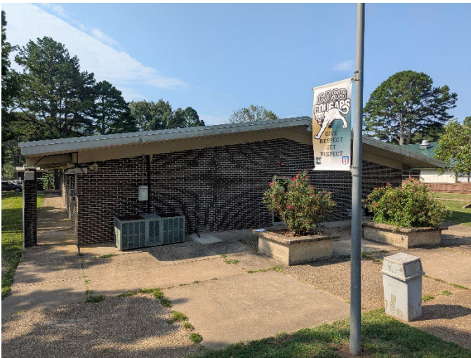
Figure 10: EDUCATION BLDG EXTERIOR AND OUTDOOR UNIT (HEAT PUMP).
