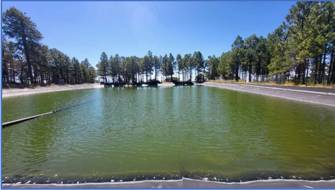
Figure 3 - Palisades Administrative Site Lagoon
