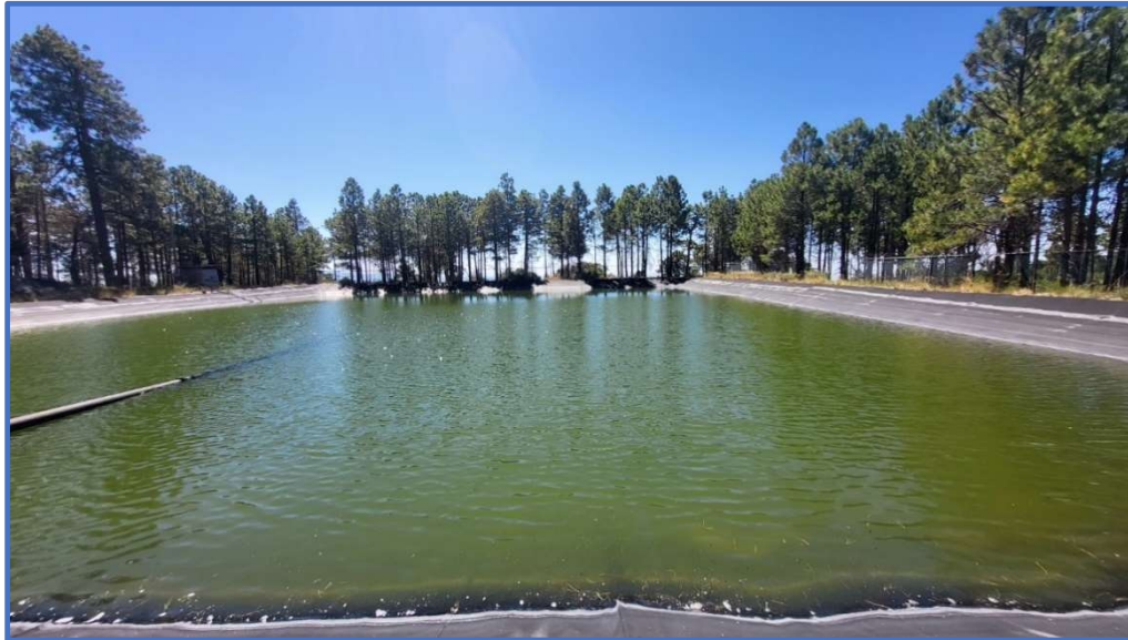
Palisades Administrative Site Lagoon (taken 9/12/2024)
