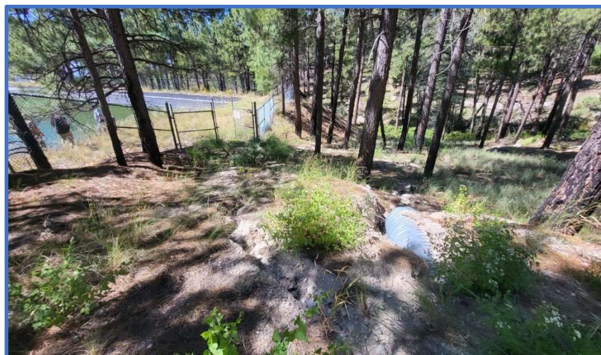
Service Access Road to Lagoon
