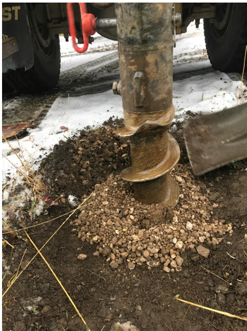
View of auger cuttings at Boring B-12
