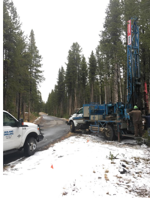
View looking north at Boring B-05
