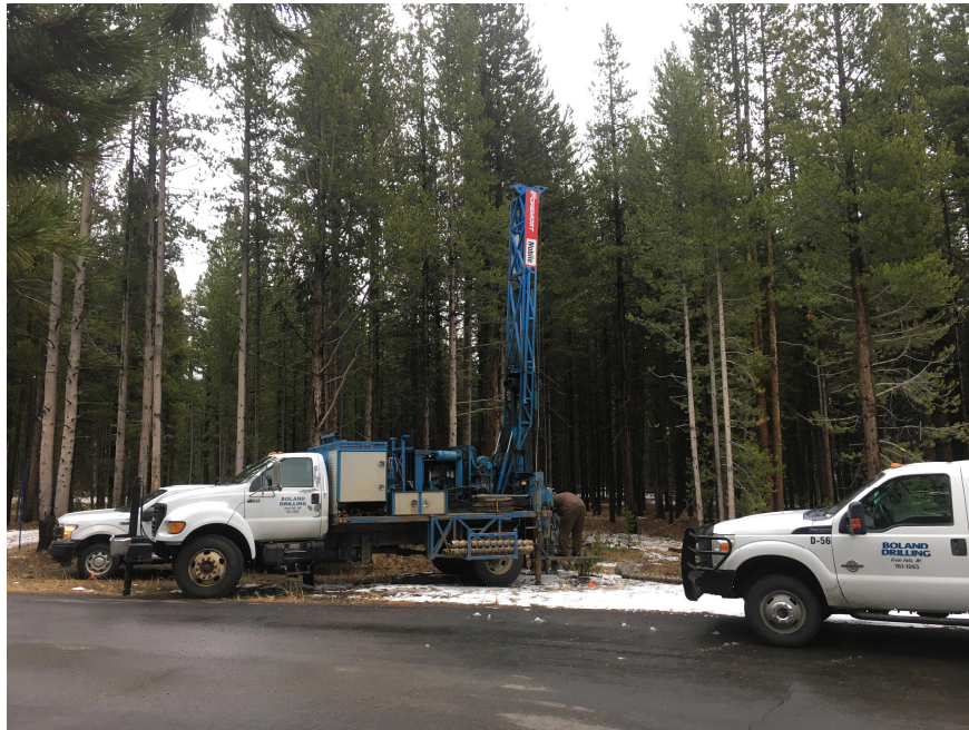
View looking east at Boring B-05
