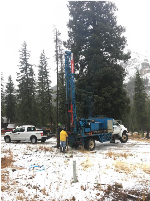
View looking south at Boring B-12
