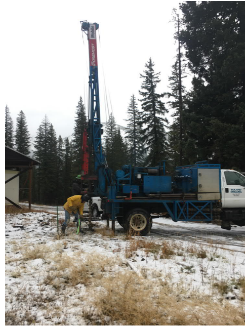
View looking east at Boring B-12
