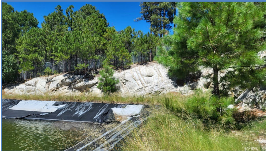
Existing Lagoon Liner – Trees and Vegetation
